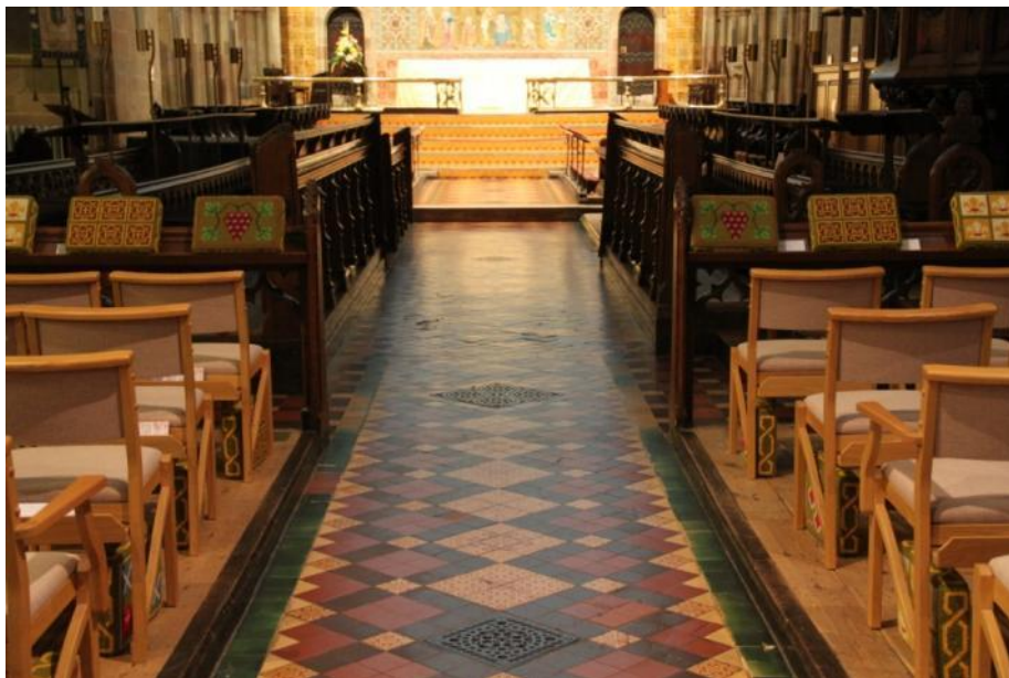
Different floor levels in the nave and chancel
