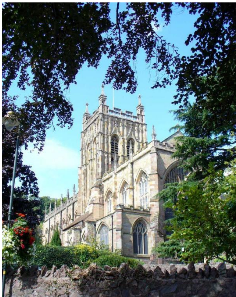
The Priory seen from the south-east (a view of the Priory from the north is shown on the front cover of the Plan)
