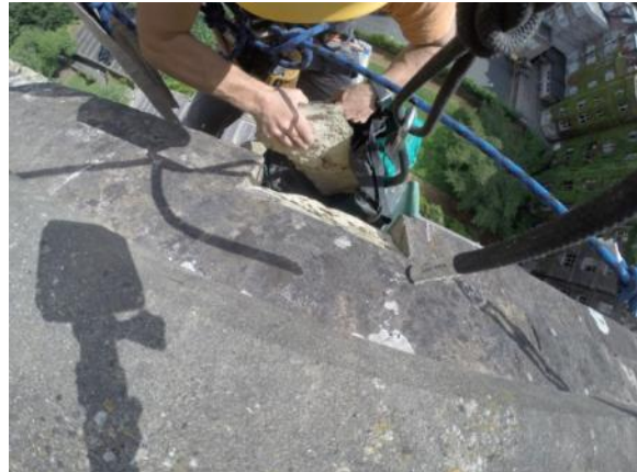
Cracked section being removed for safety
