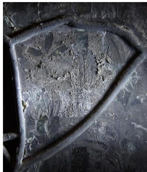
Dirt and corrosion crusts on the interior glass surface in St Anne's Chapel
