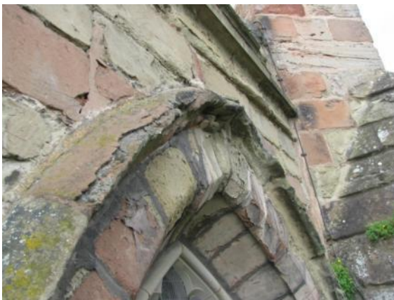
Decayed stone, failed cement pointing and vegetation bedded in open joints in exterior of St Anne's Chapel
