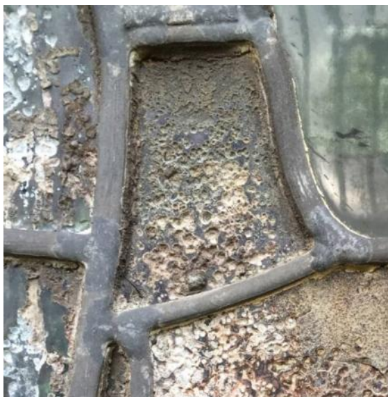
Example of corrosion from the exterior side of a window in St Anne's Chapel. Different levels of corrosion are visible, as well as extensive pitting with a mixture of dirt and corrosion products
