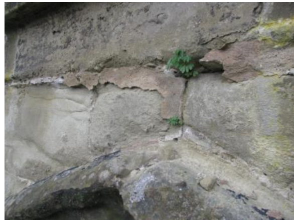
Decayed stone, failed cement pointing and vegetation bedded in open joints in exterior of St Anne's Chapel
