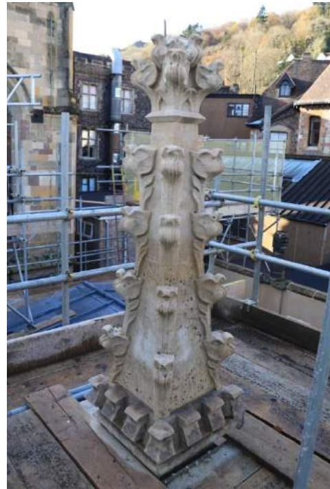
Figure 24: Left - The NW pinnacle being rebuilt (before VorTech cleaning). Right – A pinnacle after VorTech cleaning.
