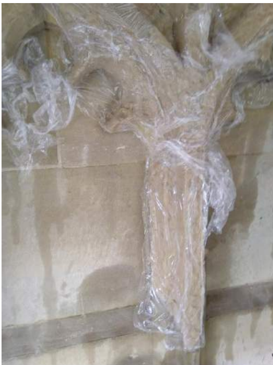
Figure 14: Ammonium carbonate poultice applied to clean carved detail.
