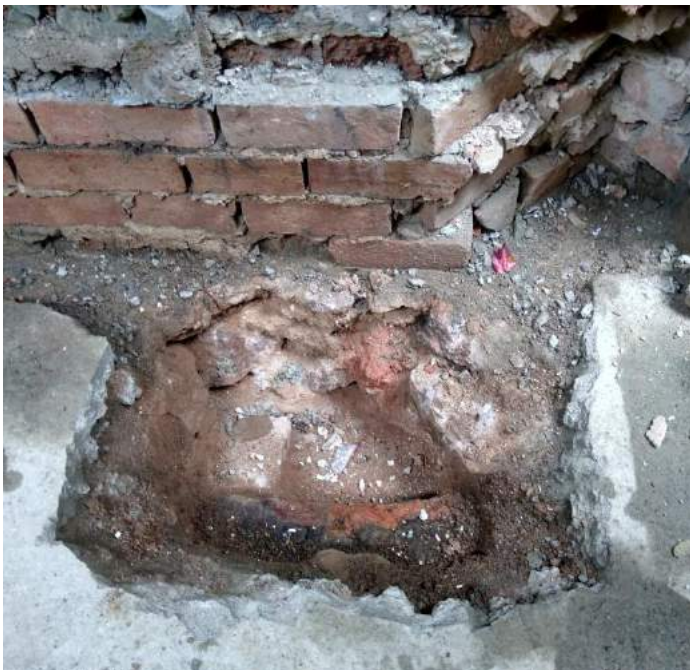
Figure 6: Trial hole dug below the level of the West Wall visible from Abbey Hotel exposing brickwork in the roof of the tunnel below
