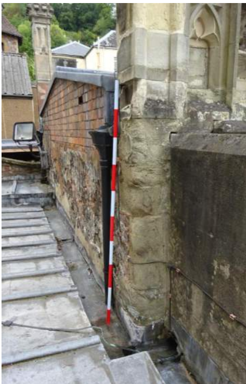
Figure 25 (left): Eroded stone at the base of the parapet under the SE pinnacle.
