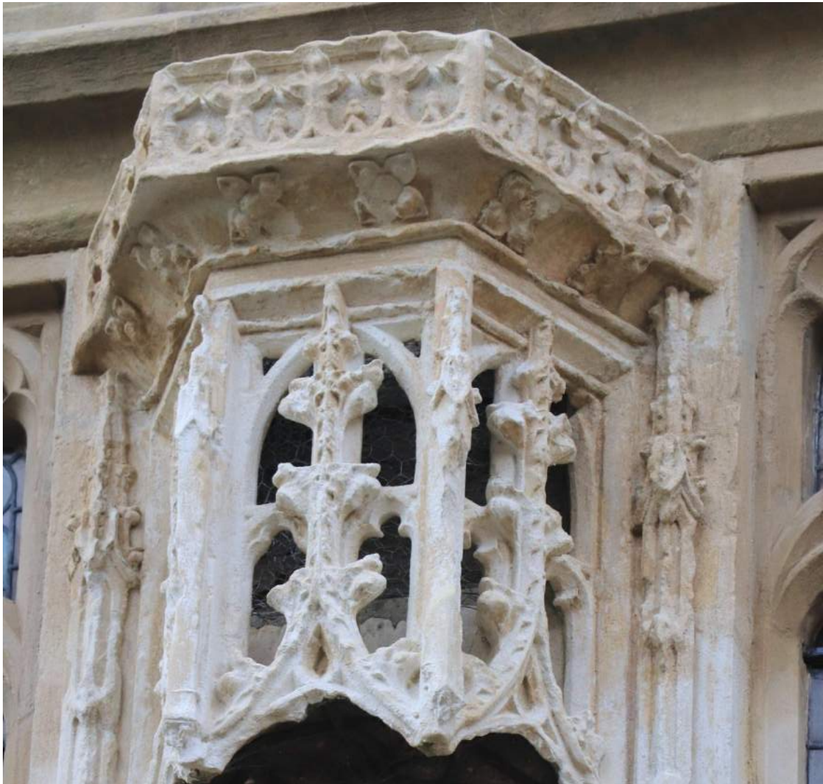
Figure 19: The cleaned and restored canopy after application of sheltercoat.
