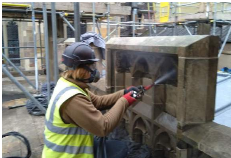
Figure 15: The VorTech machine being used to clean the stone.
