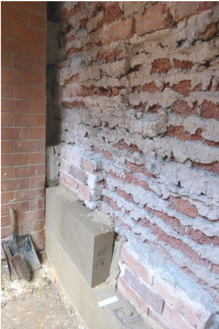
Figure 3: West Wall with stone cladding removed (Note new stone courses in place at base)
