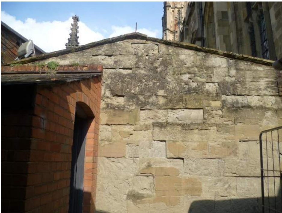
Figure 2: Section of the West Wall to be rebuilt
