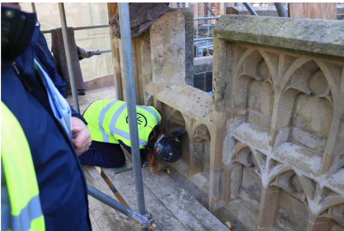
Figure 21: The section of the parapet shown in figure 20 undergoing repairs.
