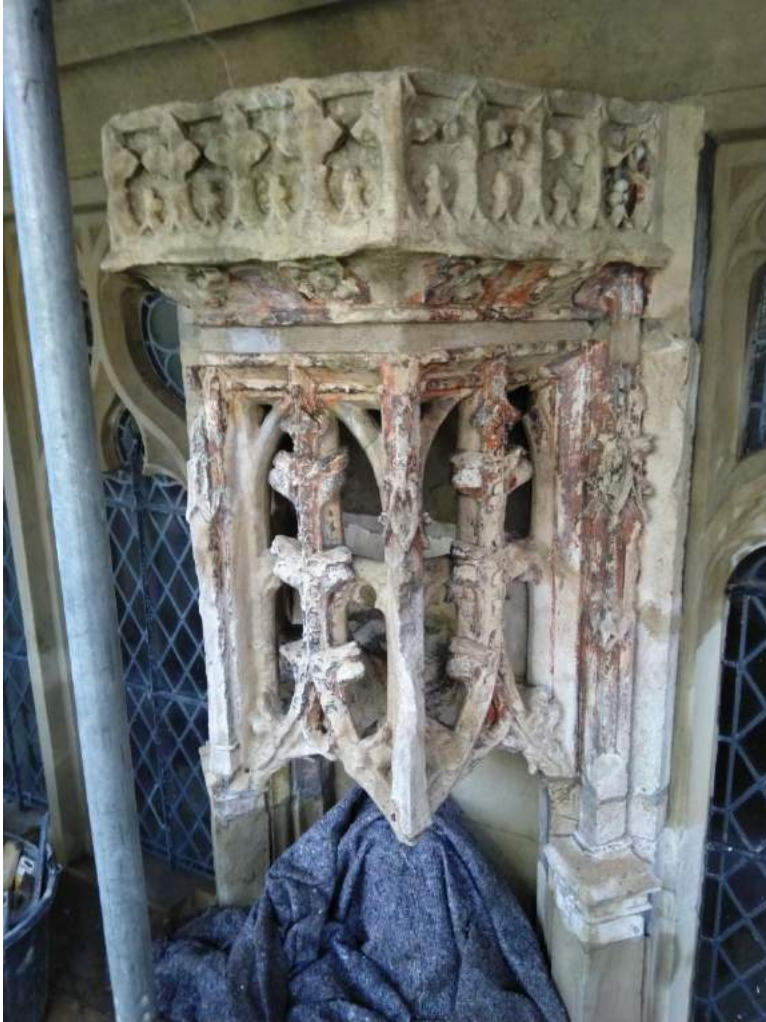
Figure 18: The canopy after removal of carbon deposits showing red paint
