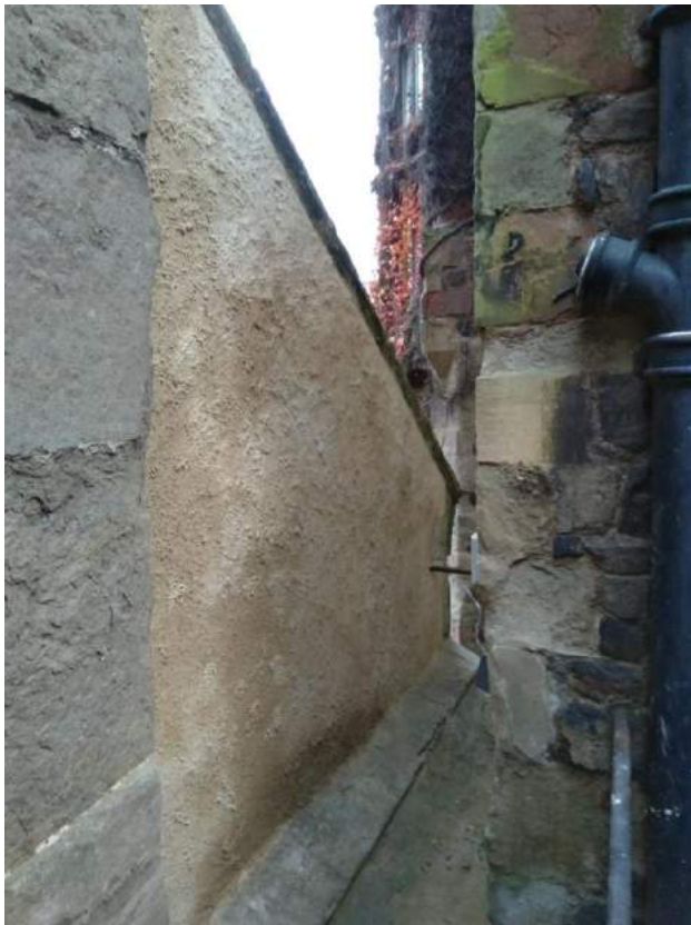
Figure 9: Completed lime roughcast render applied to S Aisle West Wall
