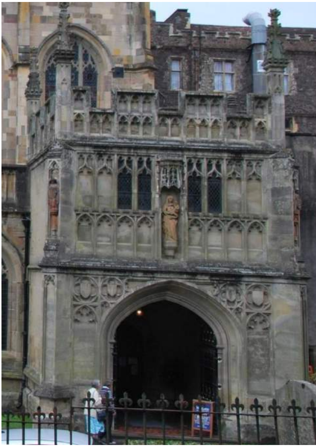
Figure 11. North Porch before work commenced.
