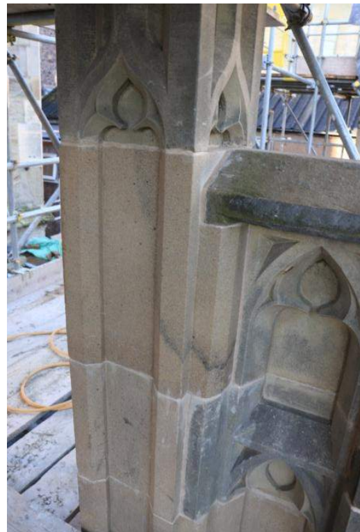
Figure 26 (right): 3 of the 4 new stones in the parapet below the SE pinnacle (the 4 th is below the scaffolding deck).
