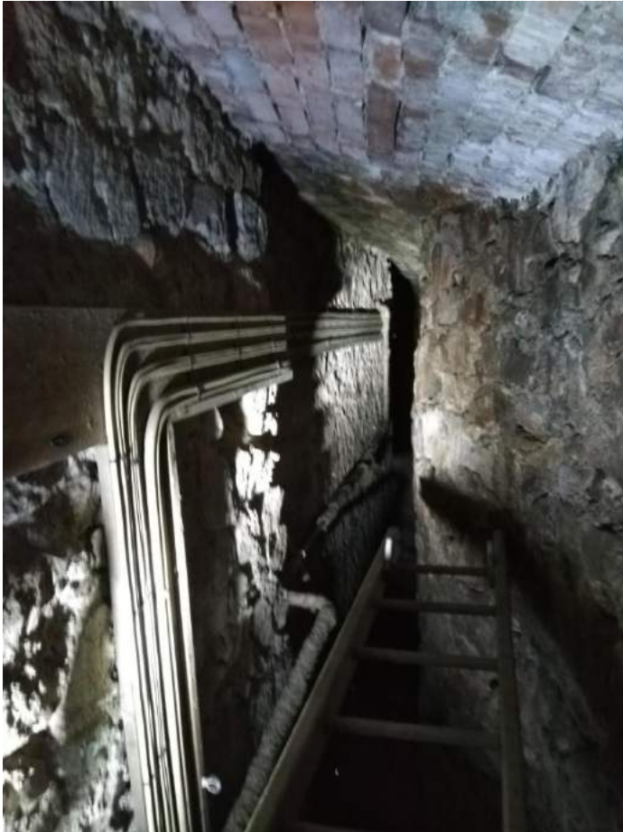
Figure 5: Interior of tunnel at north end (beyond the toilets)
