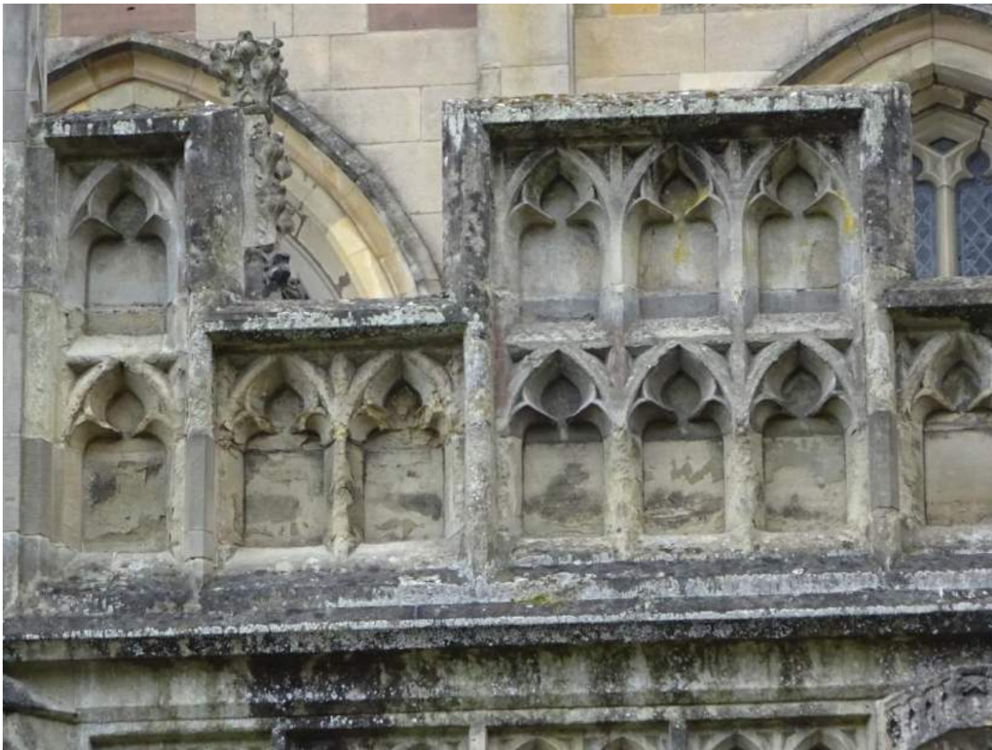
Figure 20: Original Condition of the parapet
