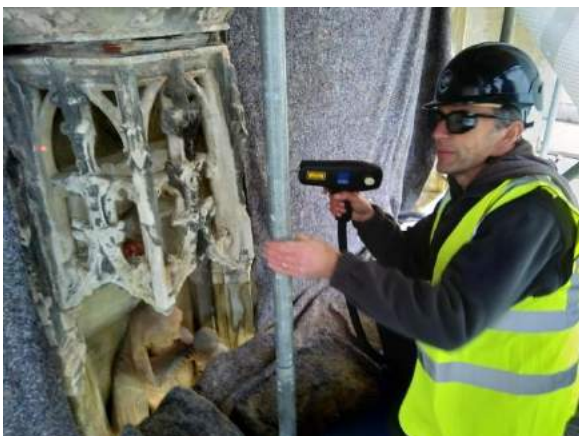
Figure 17: Laser and micro-air abrasive cleaning jet.
