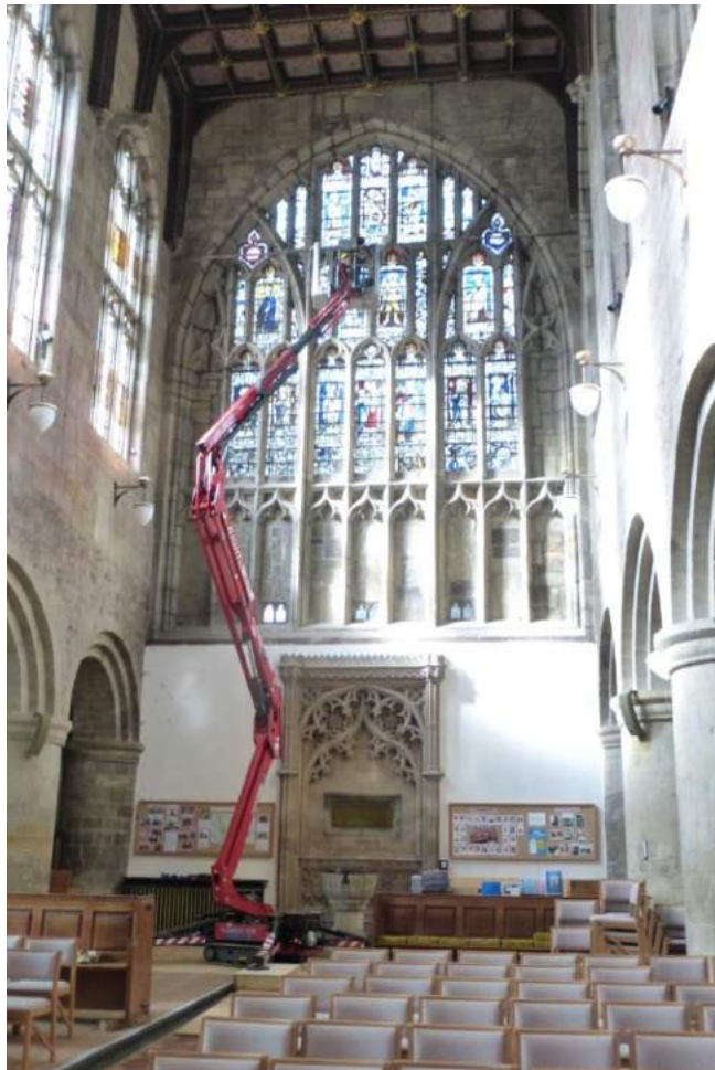
Figure 10: 'Cherry Picker' used to repoint cracks in clerestory walls.
