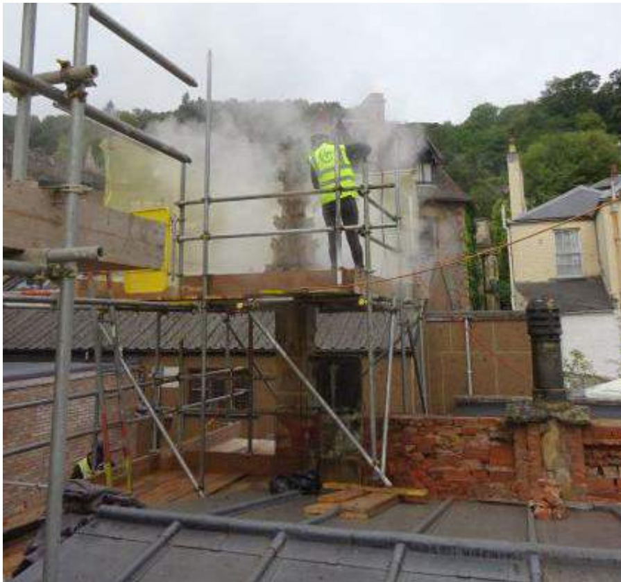
Figure 13: Stone being steam-cleaned with a ThermoTech machine.
