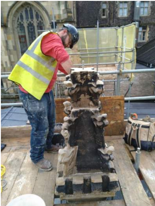
Figure 24: Left - The NW pinnacle being rebuilt (before VorTech cleaning). Right – A pinnacle after VorTech cleaning.
